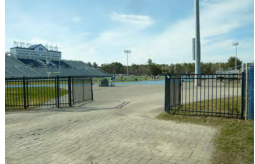
On fence at entrance with no sign
